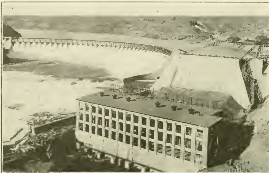
GENERAL VIEW GREAT FALLS DAM AND POWER HOUSE AT VOLTA, 4-10,000 K. W. VERTICAL GENERATORS FEED.
